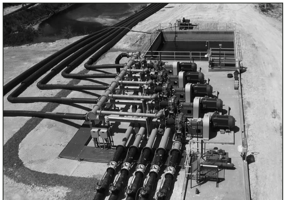
Figure 2. Goulds 8X10-29 Model 5500 Slurry Pumps in Goulds Alloy 1650 on an erosive-corrosive acid gypsum slurry transfer in Lakeland, Florida.
