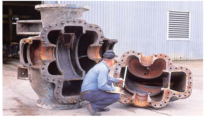
Disassembled pump is inspected for unusual wear.
