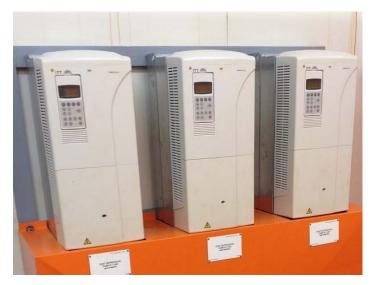
ITT PumpSmart® variable speed drive units have effectively eliminated pressure swings from the system.
